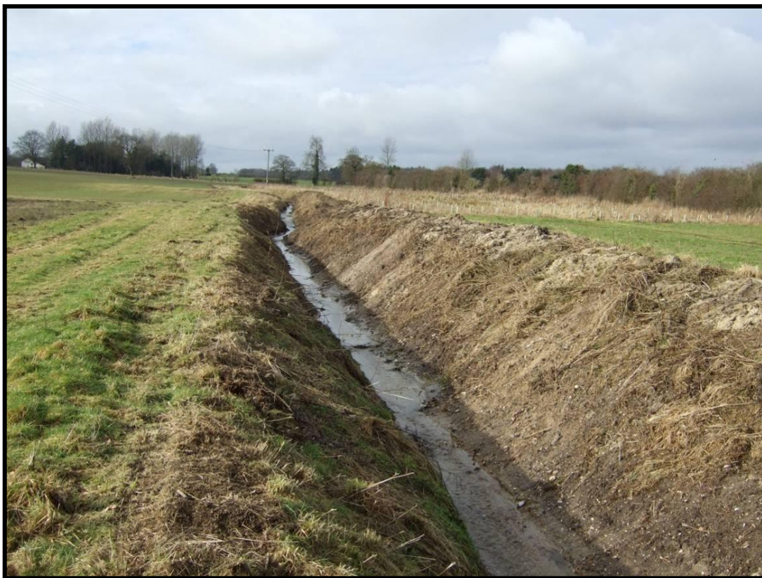
Figure 1. Resectioned bank with bare soil prone to slippage during wet weather.
