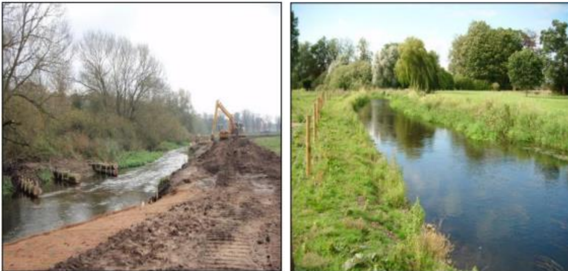
Figure 5-1. LH- Construction during November 2009, shows woody debris flow deflectors and berm creation. RH- Restored reach in August 2010. Source: EA RWRS fact sheets combined
