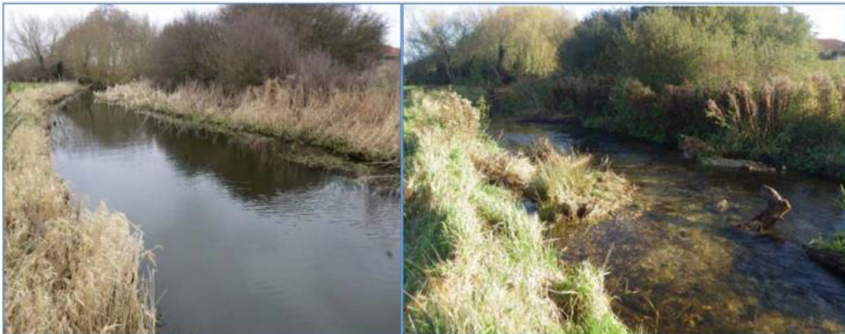
Figure 5-67. Before and after restoration photographs (Source: EA RWRS fact sheets combined)
