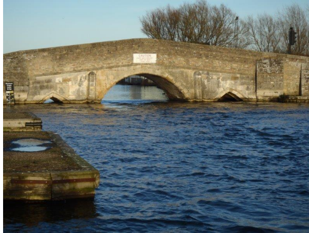
Figure 9 The medieval bridge at Potter Heigham forms an obstacle for navigation but it also considered to diminish salt intrusion in the River Thurne. Previously there has been a similar medieval bridge further downstream in the River Bure(?) at Acle. Its removal may have amplified the salt intrusion inland 1 .
