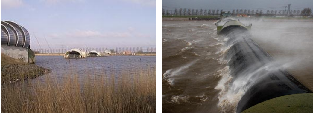
Figure 8 Inflatable rubber dam Ramspol open (left; source: nl.wikipedia.org ) and closed during storm (right; source: www.rtvoost.nl )
