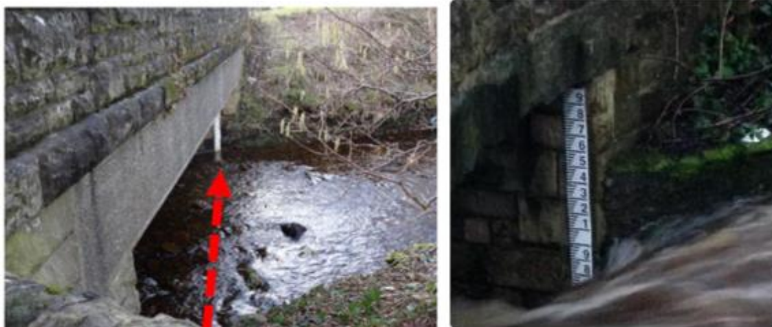
Figure E5: Gauge board positioned under a road bridge to enable observations and photos to be taken by an observer at a fixed location (Source: Starkey, 2020)
